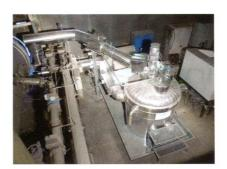
This paper deals with electric arc furnace off-gas heat recovery and first experiences with a testing plant. The testing plant based on molten salt as heat transfer fluid is installed inside the existing off-gas system of Stahlwerk Thüringen GmbH. Targets of the testing plant are to evaluate tube materials and to measure the influence of hot corrosion and dust settlement. First experimental and simulation results are presented.
